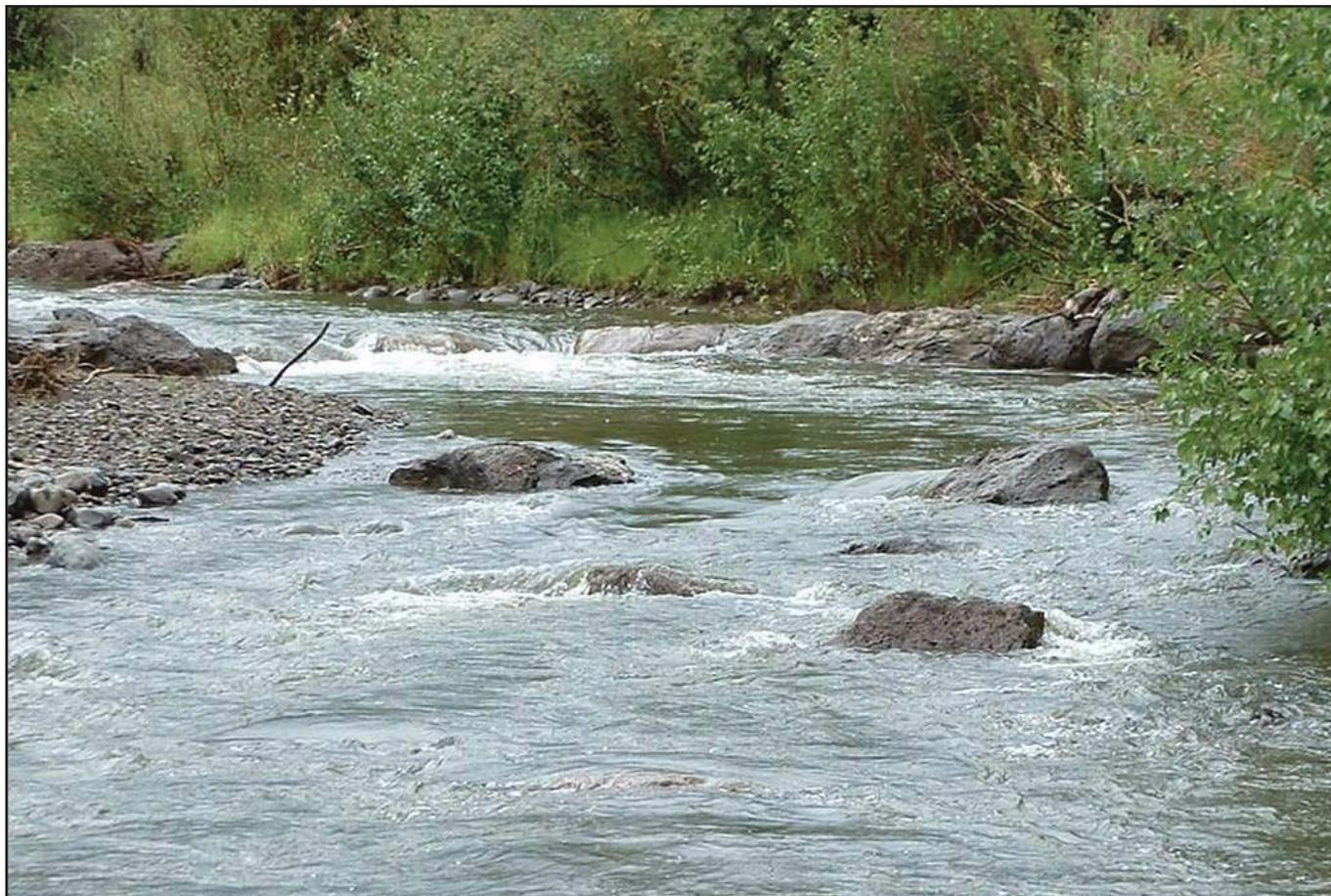
**Figure 21.** Converging rock clusters at the head of a riffle as implemented on Ohio Creek, Colorado.
