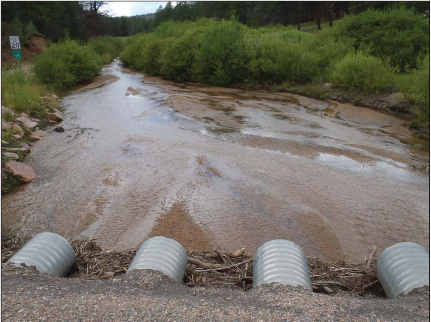
**Figure 59.** The existing stream crossing on West Creek road showing the undersized, 12" culverts and the associated, high width/depth ratio, D4 stream type (looking upstream).
