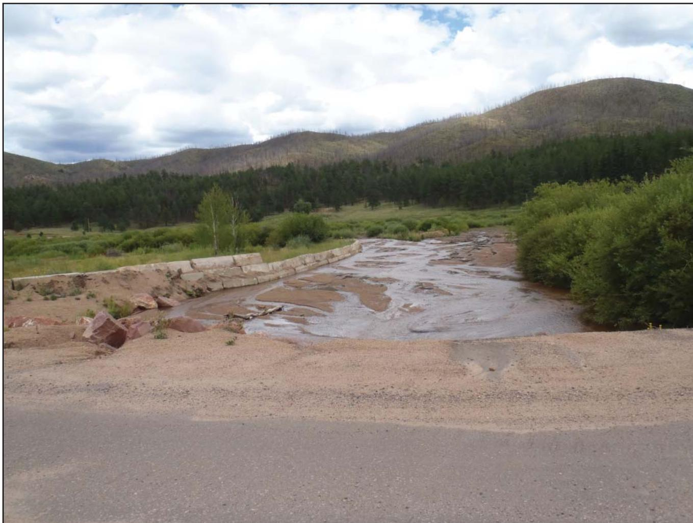
**Figure 47.** Aggradation and the corresponding D4 stream type at the mouth of Trail Creek causing flooding of adjacent landowner (note the wall on river left for flood protection).
