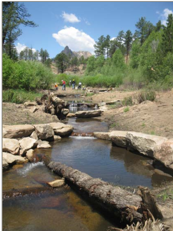
Restoration work in Trail Creek
