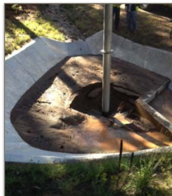
Removal of 8 cubic yards of sediment using a vacuum truck along Sugar Creek
