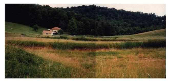
Note the following features of this system. The wetlands are *integrated* within the landscape: looking at them, you wouldn't know they're acting as treatment systems for mine drainage. Several wetlands are used for treatment, rather than a single one. This is due to restrictions imposed by the landscape and the need to achieve a specified surface area for treatment. Furthermore, their elongated shape maximizes contact between the water and the wetland surface.
